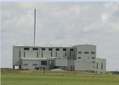
The flue gas treatment process at this Energy from Waste plant in Grimsby uses hydrated lime which reduces acid gas emissions such as hydrochloric and sulphuric acids by turning them into harmless solid calcium salts.
