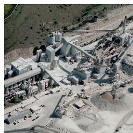
There are two main types of lime and both are produced by burning rock at high temperatures in a kiln. High calcium lime is made from burning limestone or chalk, which is chemically known as calcium carbonate ( $\text{CaCO}_3$ ) at temperatures of up to  $1000^\circ\text{C}$  in either a vertical or horizontal kiln. Dolomitic lime is made from burning limestone and
