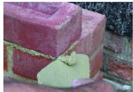
(calcium carbonate). The crystals formed by this process help to plug the hairline cracks.
